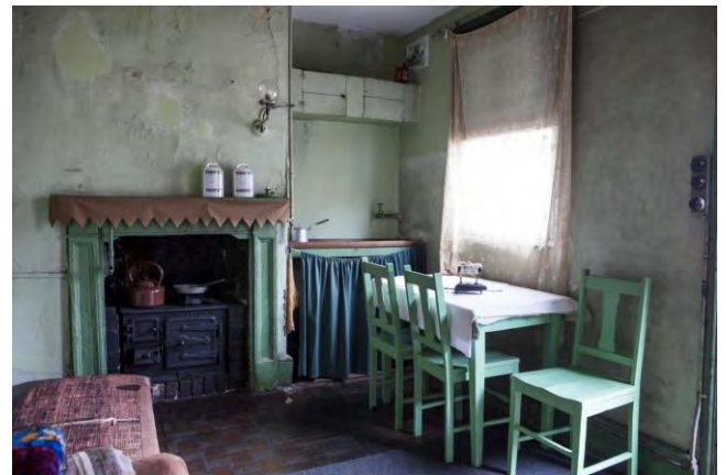
The kitchen at 60 Gloucester Street, The Rocks, as seen today in Susannah Place Museum, representing the Sarantides’ occupation in the 1930s and 40s © James Horan for Sydney Living Museums
