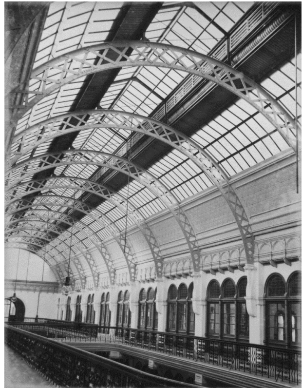
Interior view from the upper (retail) level of the Queen Victoria Building immediately prior to its opening, 1893.
